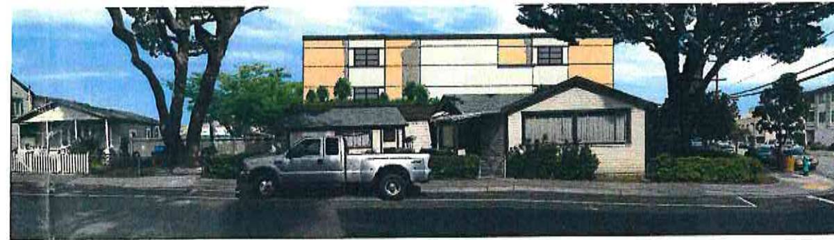
2 VIEW FROM MARIPOSA STREET
